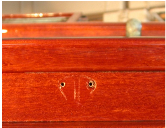
B: Without hardware showing difference between exposed wood and non exposed wood.
